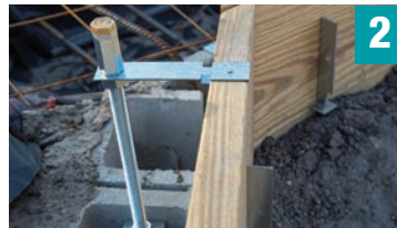
Tack Anchor Bolt Assemblies at each location
