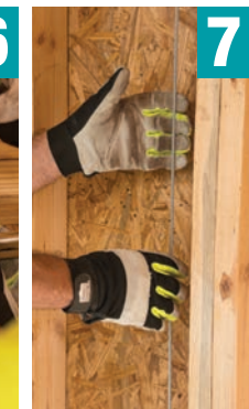
7 Check the tension on the installed cables
