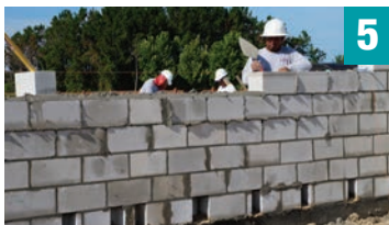
Finish laying CMU block wall in running bond pattern
