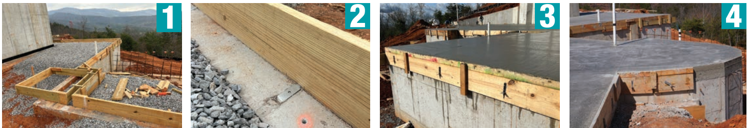
Concrete slab formwork w/ Form Ties
