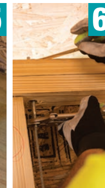
6 Tighten QuickTie™ at top plate
